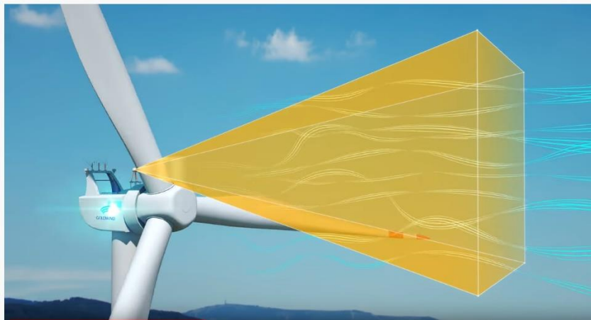
Goldwind's EFarm optimizes operation by the use of lidar-assisted control.
